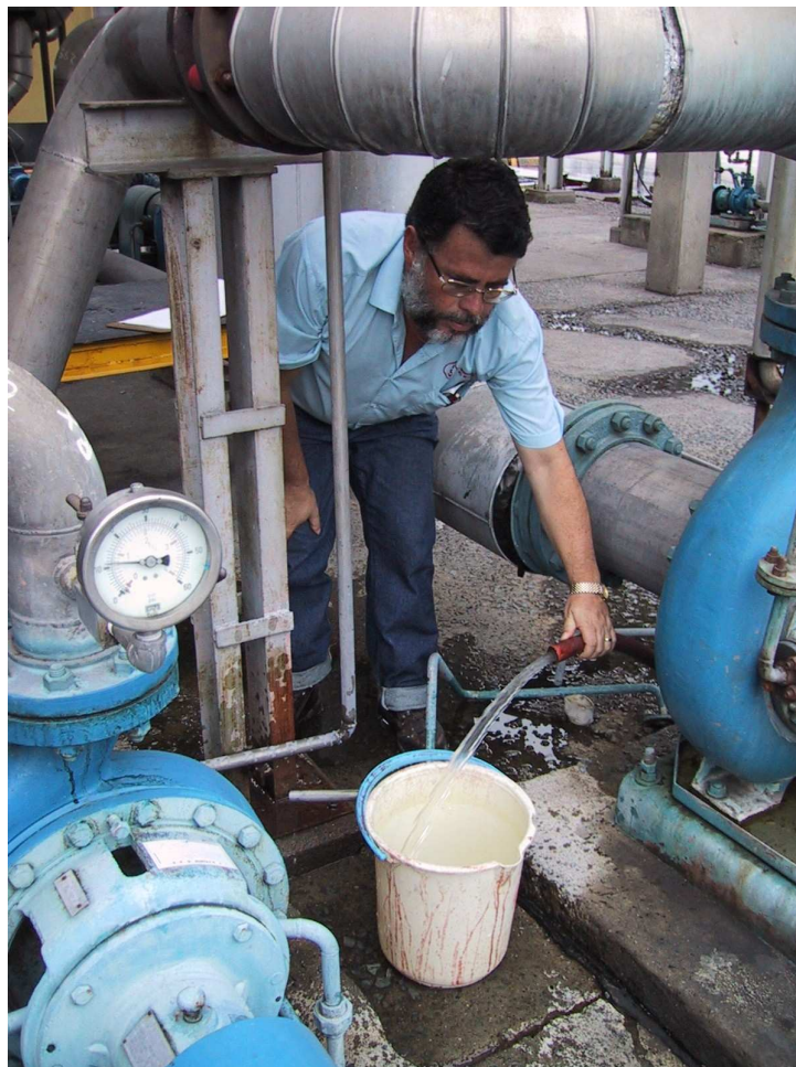
Figure 1: The “bucket engineer”
